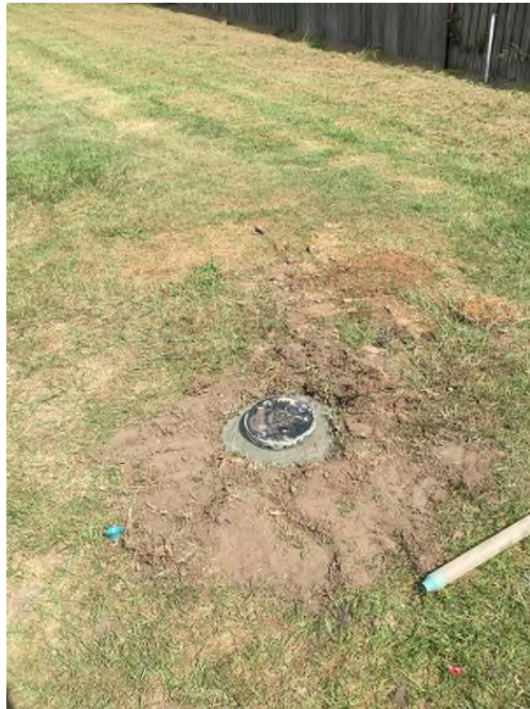
Photograph 7. Monitoring well MW01 installed and developed on 7 November.
