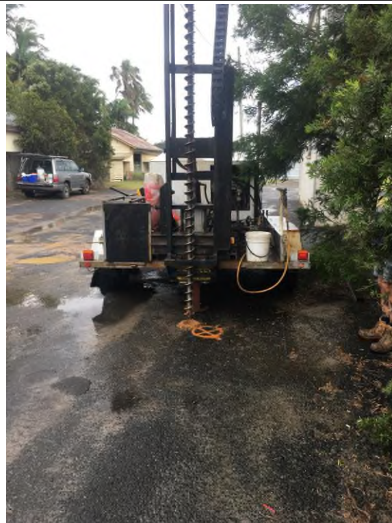
Photograph 8. Soil boring location SB07 with ~ 30mm of asphalt at the surface.
